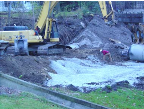
Construction taking place at Allen Park
