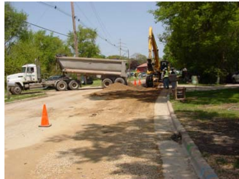
Construction taking place at Champlain Street sanitary sewer
