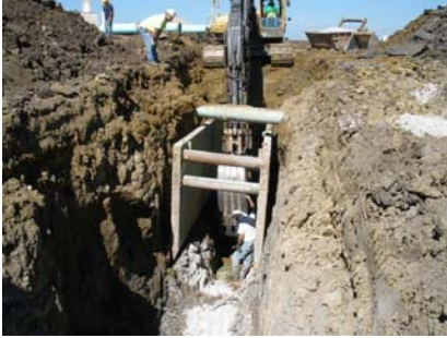
Water main extension to Kohl's Distribution
