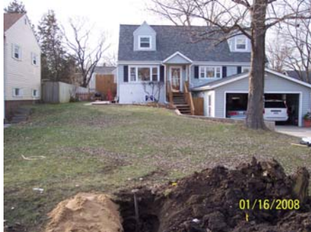
Parks Lane Water main extension
