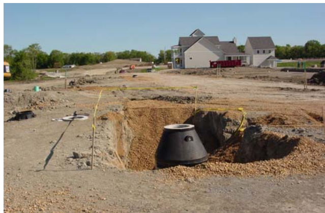
Sanitary sewer construction to Heritage Harbor Ottawa
