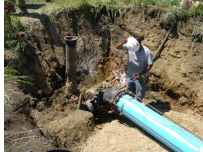
Water main extension on MBL Drive
