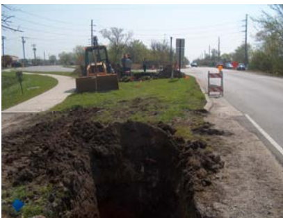
Water main extension to Heritage Harbor
