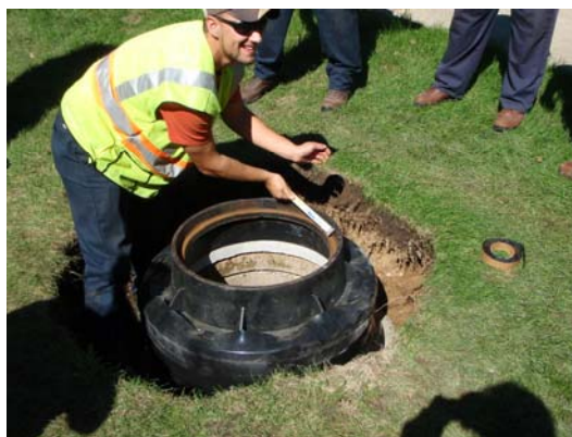
Staff installing chimney seal during a training session
